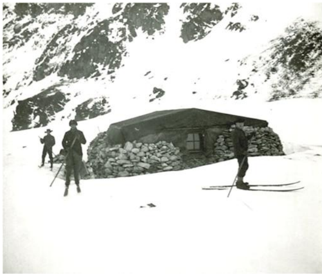
Above: photograph of the newly completed Omond House with its original ‘sailcloth’ roof, and three unnamed crew on perhaps an early attempt at skiing with a single pole each. Photograph courtesy of the Estate of William A. Cuthbertson
